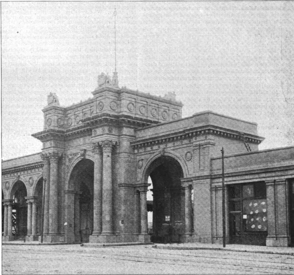
Fig. 1.—High-Street Entrance to Union Passenger Station, Columbus, Ohio.
